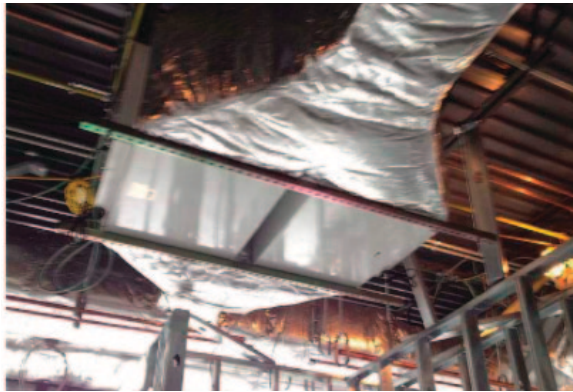
Two units were bundled to purify the air in this IVF lab in Chapel Hill, NC.
